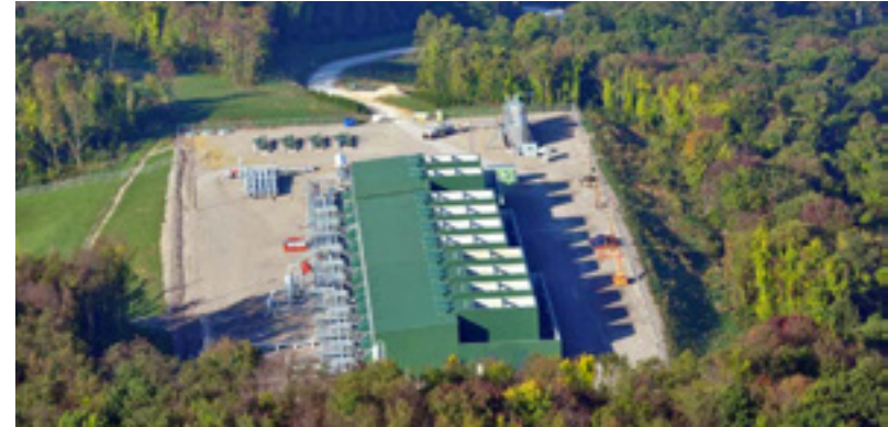
Three Brothers Compressor Station, PA. By Bob Donnan, 2014
