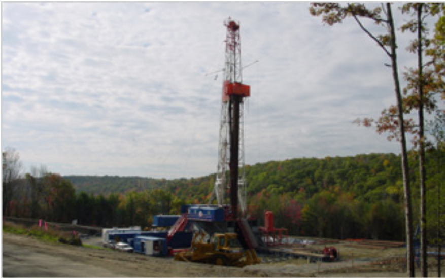
A partially reclaimed single-well site in Chemung County, New York. The footprint of the drill site was 3.2 acres, reduced to a fenced area of 0.45 acres. Photo credits: Henkel, 2002 and 2009. Used with permission. Source: NY Draft SGEIS 2011, p. 6-336.
