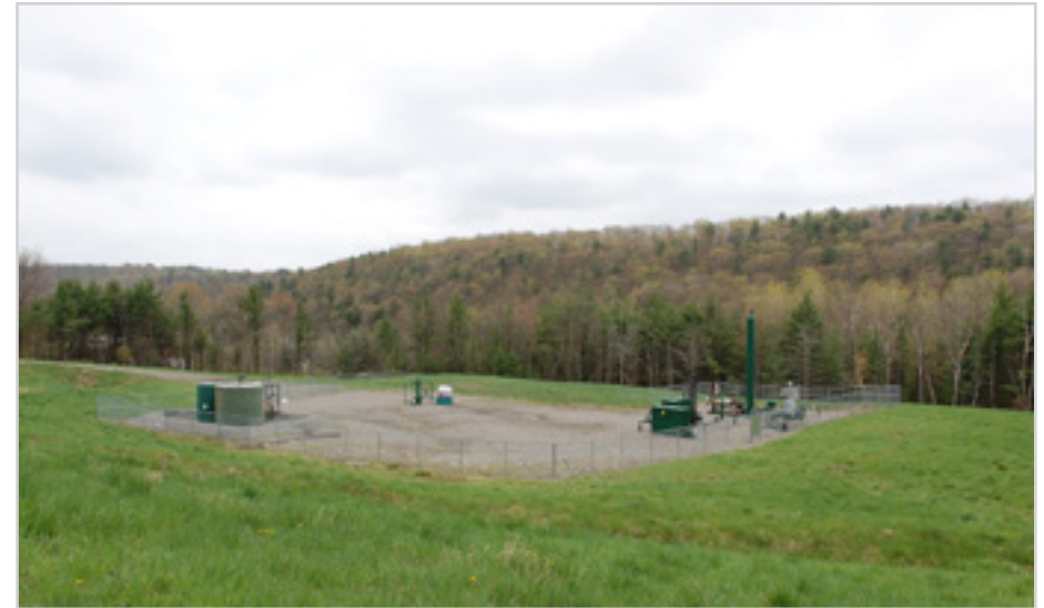
A partially reclaimed single-well site in Chemung County, New York. The footprint of the drill site was 3.2 acres, reduced to a fenced area of 0.45 acres. Photo credits: Henkel, 2002 and 2009. Used with permission. Source: NY Draft SGEIS 2011, p. 6-336.
