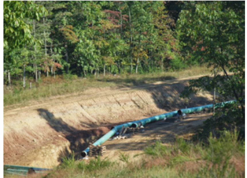
Pipeline under construction in WV. By Samantha Malone 2013.
