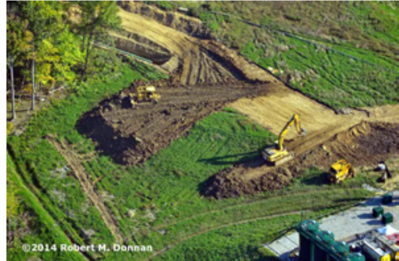
Gathering pipeline construction, PA. Photo by Bob Donnan, 2014.
