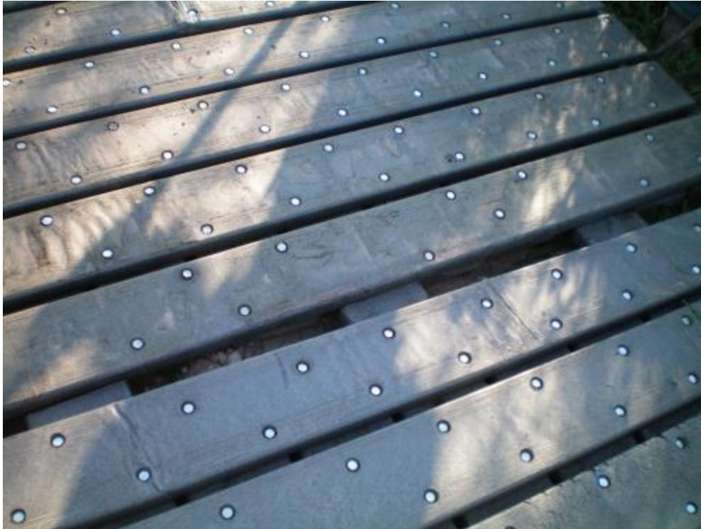
Figure 16. Top view of tongue and groove connections between two Wyoming Flat panels.
