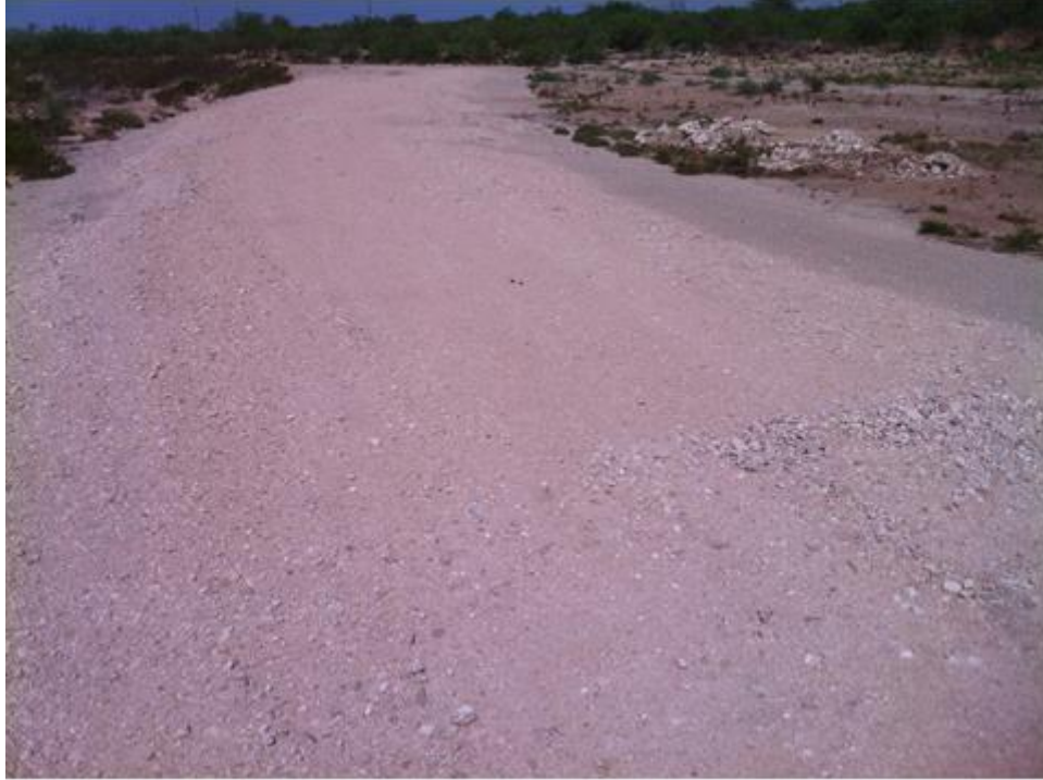
Figure 43. Spine road using well cutting after two years. Note no growth of plant life and limited weather wear on road section.
