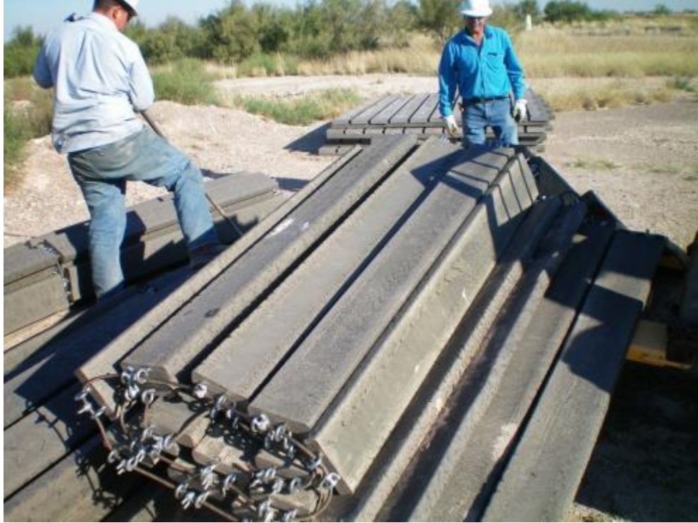
Figure 20. Stored Wyoming Roll-out mats after unloading from truck.
