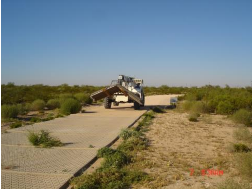
Figure 22. Movement of Wyoming Roll out panels can be difficult due the inability of the mats to lie flat on the forklift with the connection between panels.
