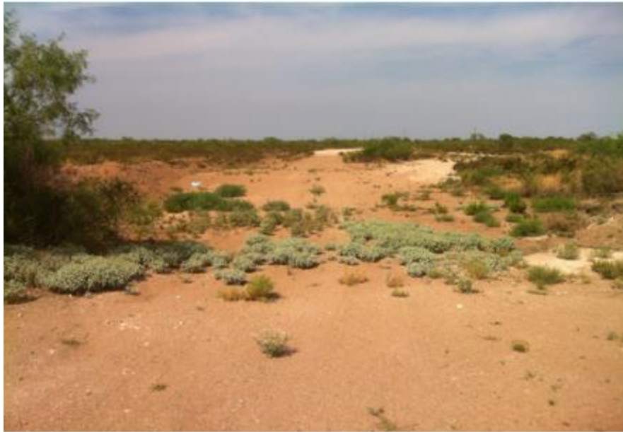
Figure 39. View of temporary road from track towards interior of facility. Note return of weeds and plant life to roadbed. Roadbed has been graded in last 4 months in preparations for a permanent road.
