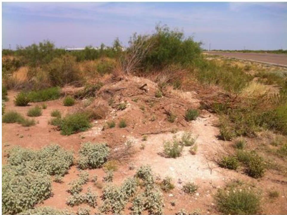
Figure 42. Are to side of roadbed that has been cleared for future work.
