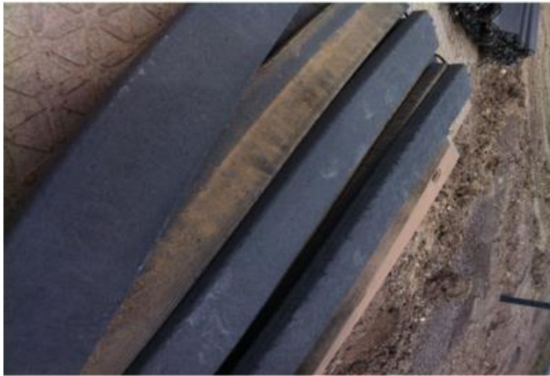
Figure 48. Due to the overlap of the Newpark mats some type of support needed for the overlap section of the mats. Each mat is made of two panels with an approximate offset of 8 inches in two directions of the panels. Without a specific trim piece for this section alternative methods are required to support the edge of the mats.
