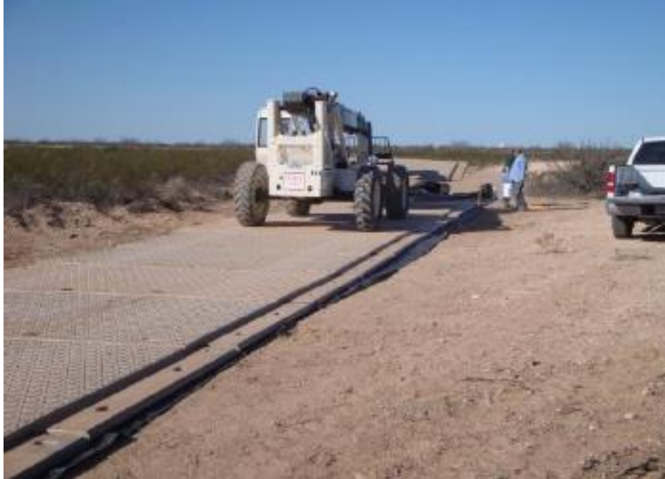
Figure 8 Newpark mat installation at Pecos Test Site.
