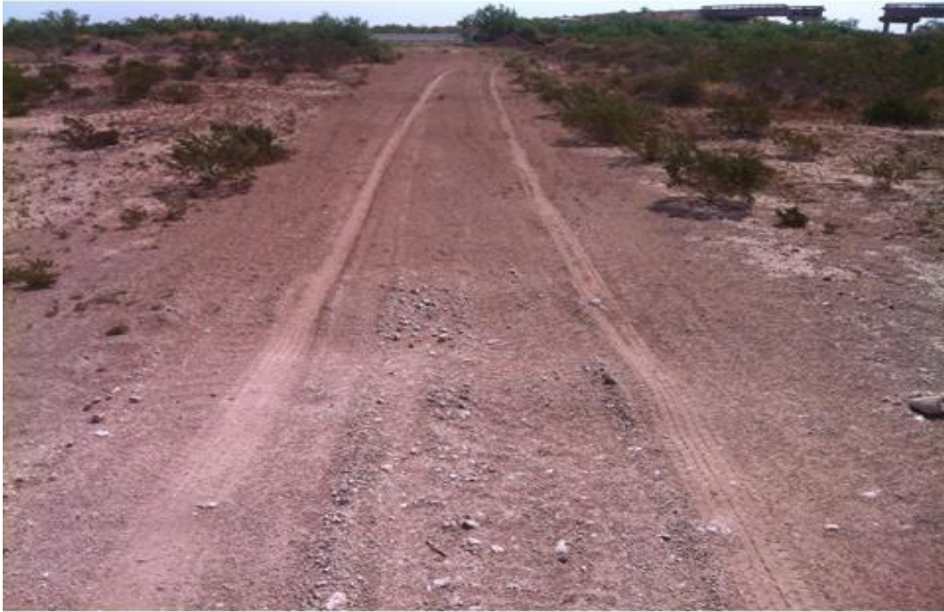
Figure 41. Reverse view of road from spline road section to Track. Note tilled soft dirt versus hard packed caliche. Material will allow for growth of plant life on old road.
