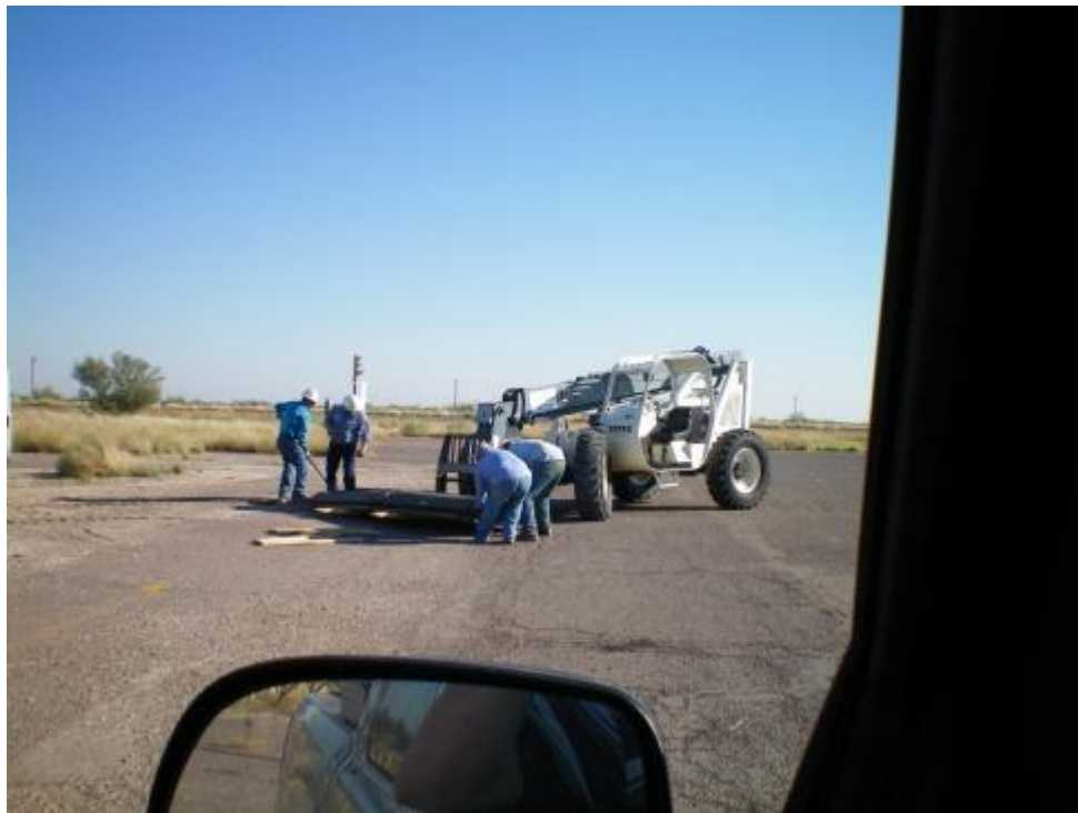
Figure 21. Wyoming Rollout panels must be rolled out and unfolded after shipment. All panels were packed this way to save space during shipment.
