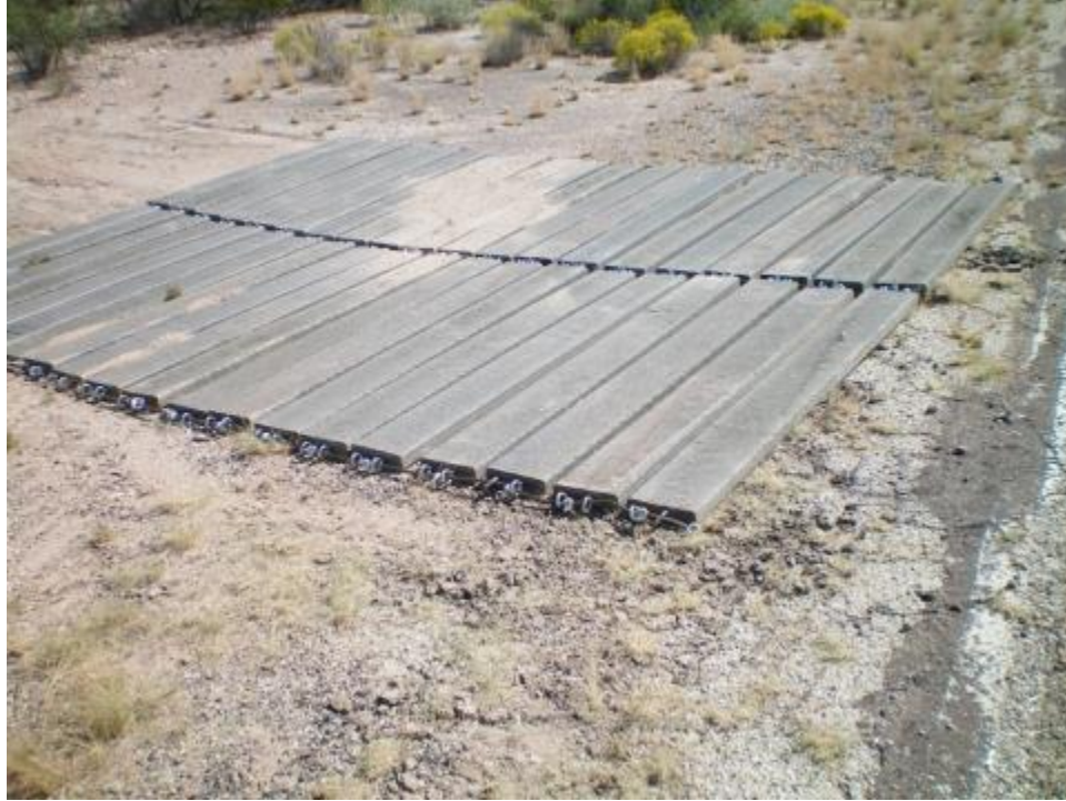
Figure 33. Wyoming Roll out panel as installed from roadway note flat installation before twist of panel to match street intersection.
