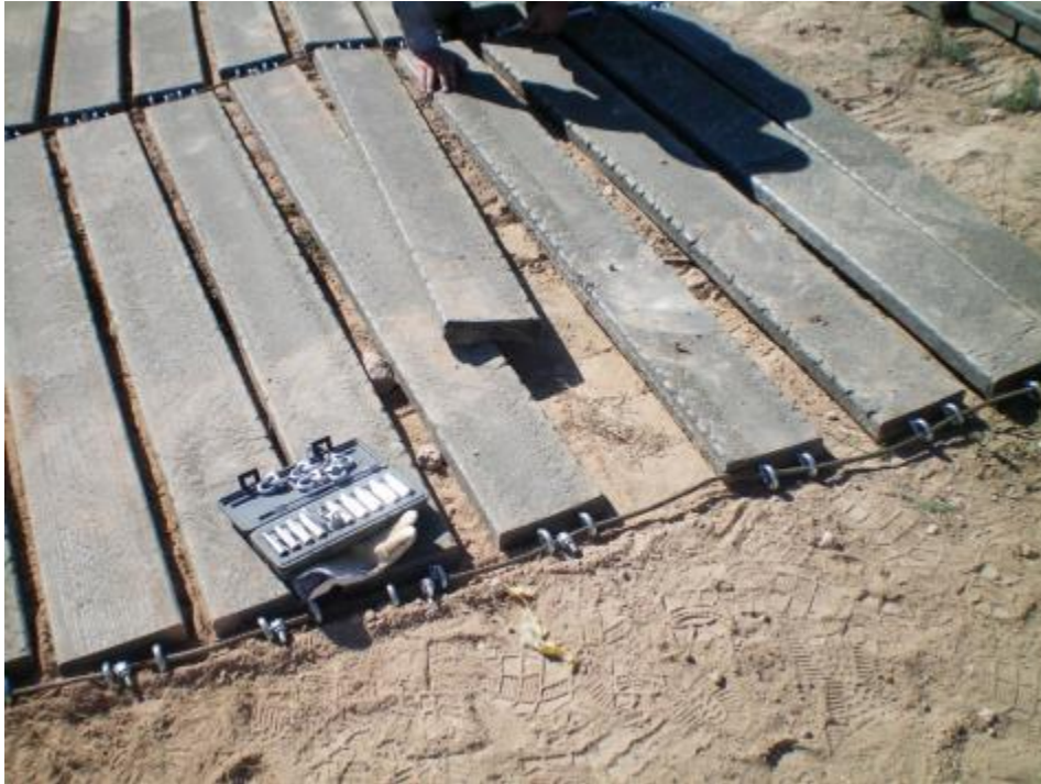
Figure 26. Removal of broken interior board of Wyoming rollout mat.
