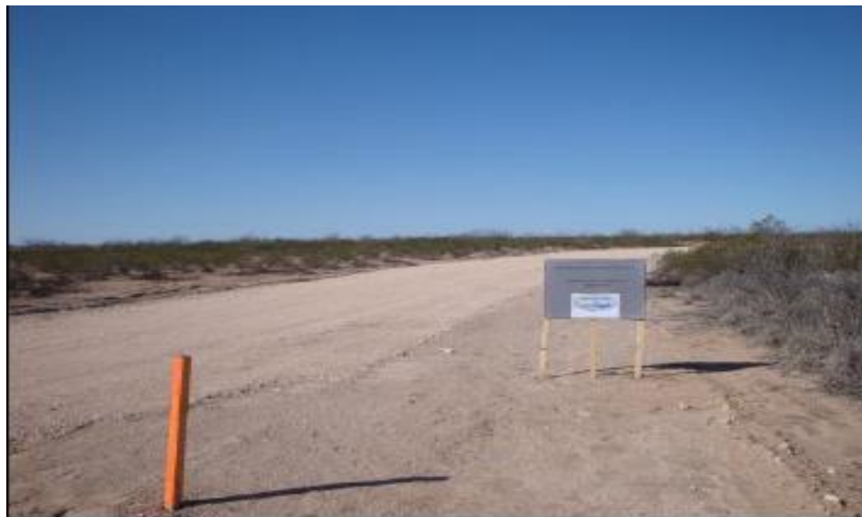
Figure 7. Completed Spine Road Section
