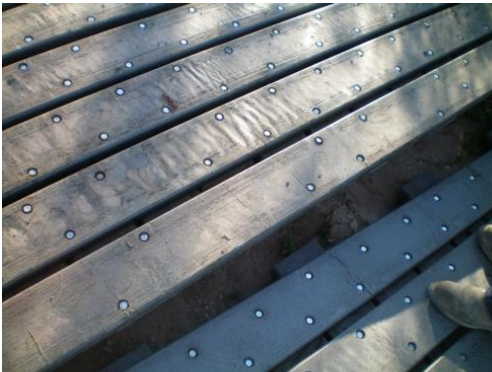
Figure 15. Adjustments required to match two panels to finalize installation of panels.
