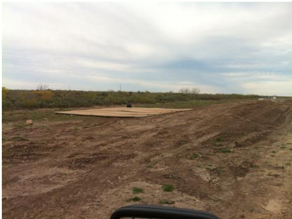
Figure 54. Final layout of pad behind production facility.
