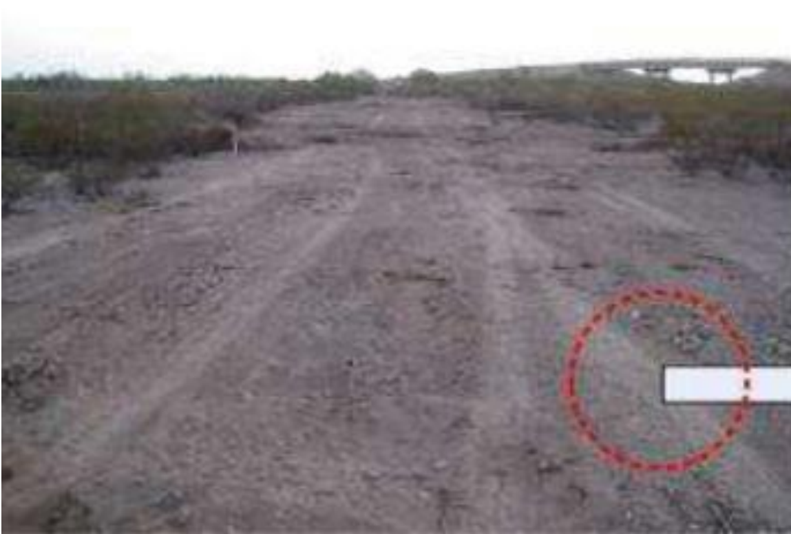
Figure 4. Photograph of dirt road to be used for spine section of test. Note overpass has not been removed from entry road.
