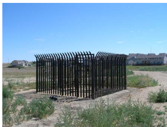
Typically, fencing around well heads or tank batteries consists of chain link and razor wire. This alternative fencing meets industry safety standards and matches the character of the neighborhood. Courtesy of Todd Tucker, Town of Frederick.
